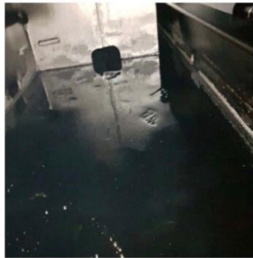
TANK INSIDE WITH REMAINING OIL
